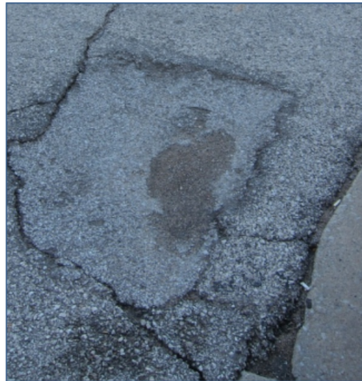
Poor roadway conditions in the project area will be reconstructed
