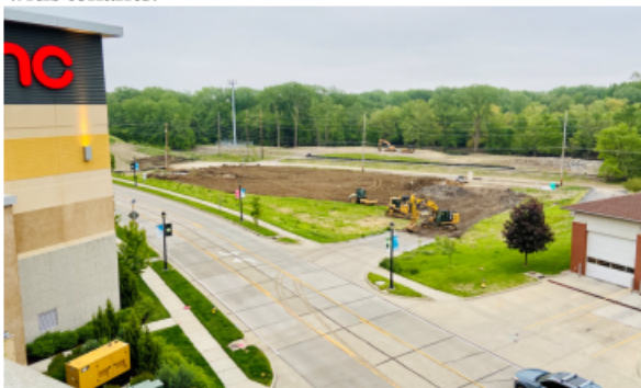
Utility work and grading is underway at Phase 1 of the project
